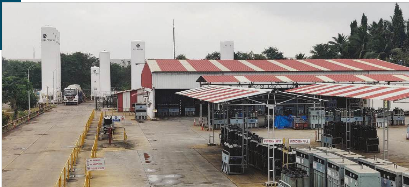
Aerial View of an AWIPL state-of-the-art Filling Station.
